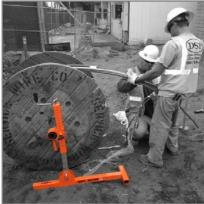
Separate sides can be used safely on uneven ground
