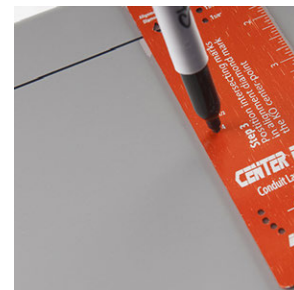
4. Mark the center of the hole
