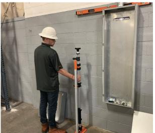
Step 4: On lower pin, pull pin to adjust rough height of final position and reengage within 12 to 15 inches below the final anchored position of the workpiece.
